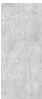
R109 Concrete, PT
